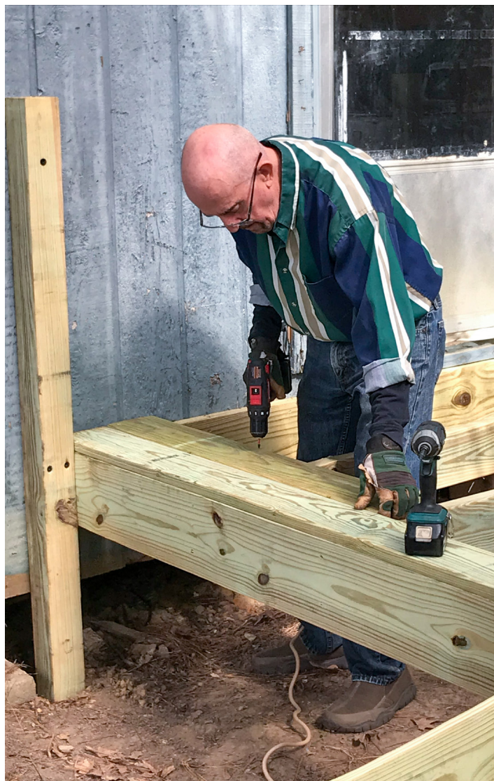
Members of Sylvan Hills UMC's United Methodist Men recently built a wheelchair ramp for a former nursery supervisor at the church. The group is intergenerational, making it unique compared to many other UMM groups. || Photo provided by Sylvan Hills UMC
