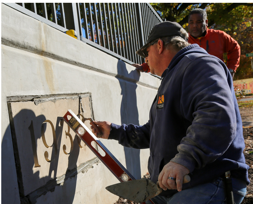
Facilities Supervisor Dan Guido installs the original 1936 cornerstone into the new handicap accessible chapel entry. || Photo by Lori Krie
