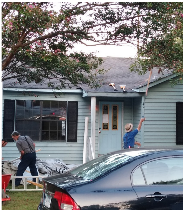
Top: Christian Aid Ministries partners with the Arkansas Conference to build roofs for homes.
