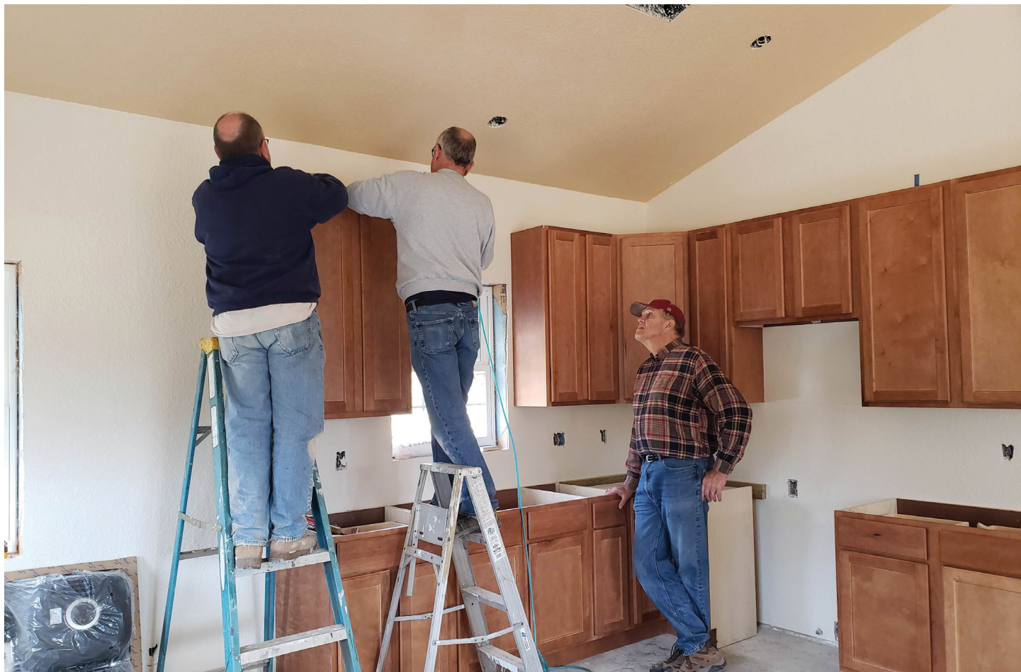
A recovery team from Roger's FUMC installs cabinets in a rebuilt home that was destroyed in the April 2018 Crawford County Tornado.
