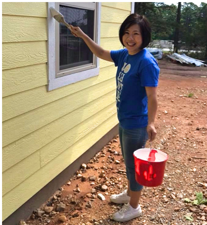
A volunteer paints the outside of one of the ECHO Village homes.
