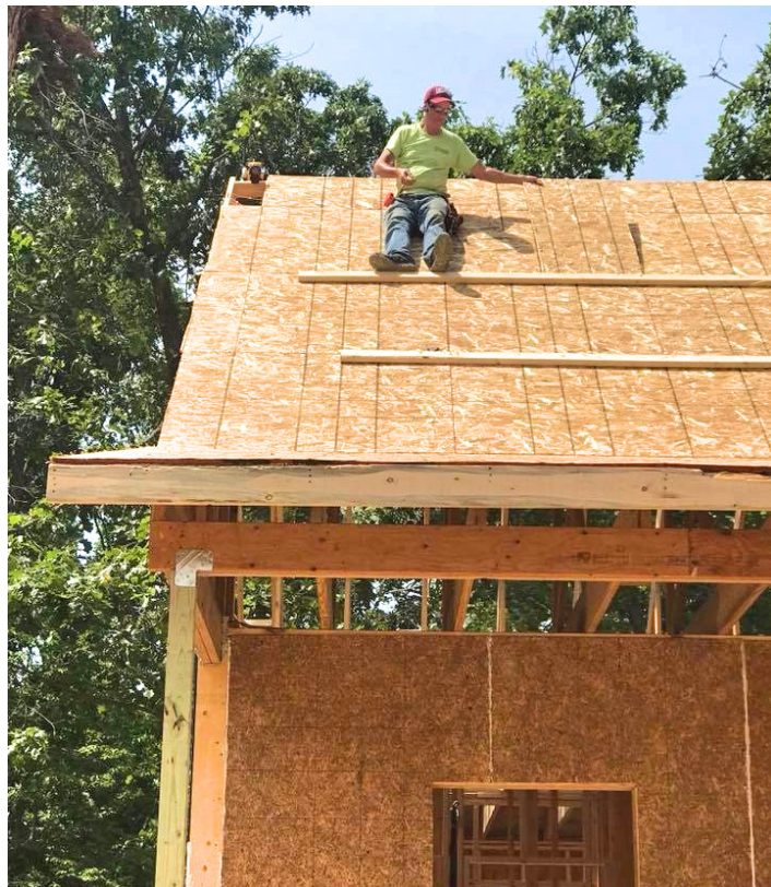
A volunteer sits on top of one of the homes to help assemble the roof of a new house in ECHO Village.
