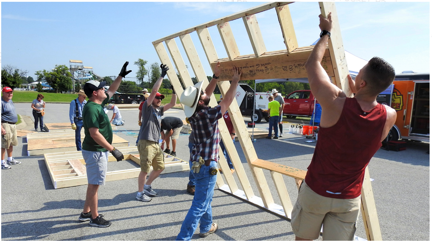
Volunteers lift one of the interior walls built during the build weekend in Rogers, Arkansas. Volunteers were encourage to write Bible verses or words of encouragements on the boards of the walls that were assembled. In all, 40 interior and exterior walls were assembled on Aug. 11.
