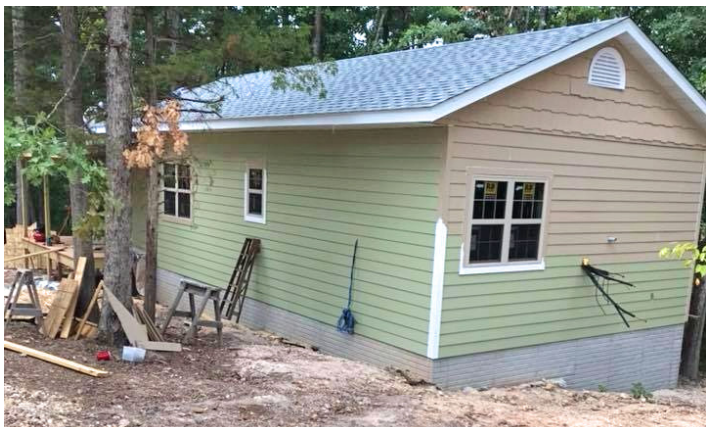
A volunteer paints the outside of one of the ECHO Village homes.
