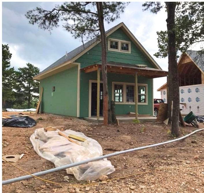
One of the eight houses in ECHO Village sits nearly complete on a 10-acre plot of land in Eureka Springs, Arkansas.
