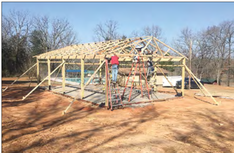
Construction of a new pavilion at Shoal Creek Camp is under way. The structure should be completed in time for this summer’s camps, which begin with the June 28 Big Apple younger elementary camp.
