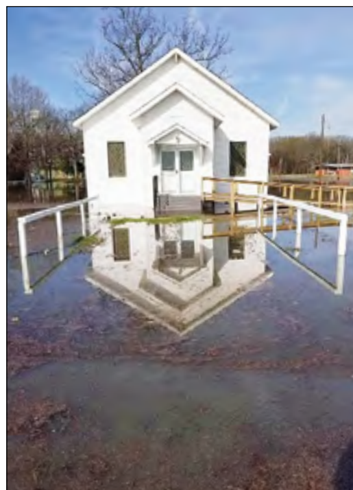
After a levee breach, water surrounds Humnoke United Methodist Church on March 9.
