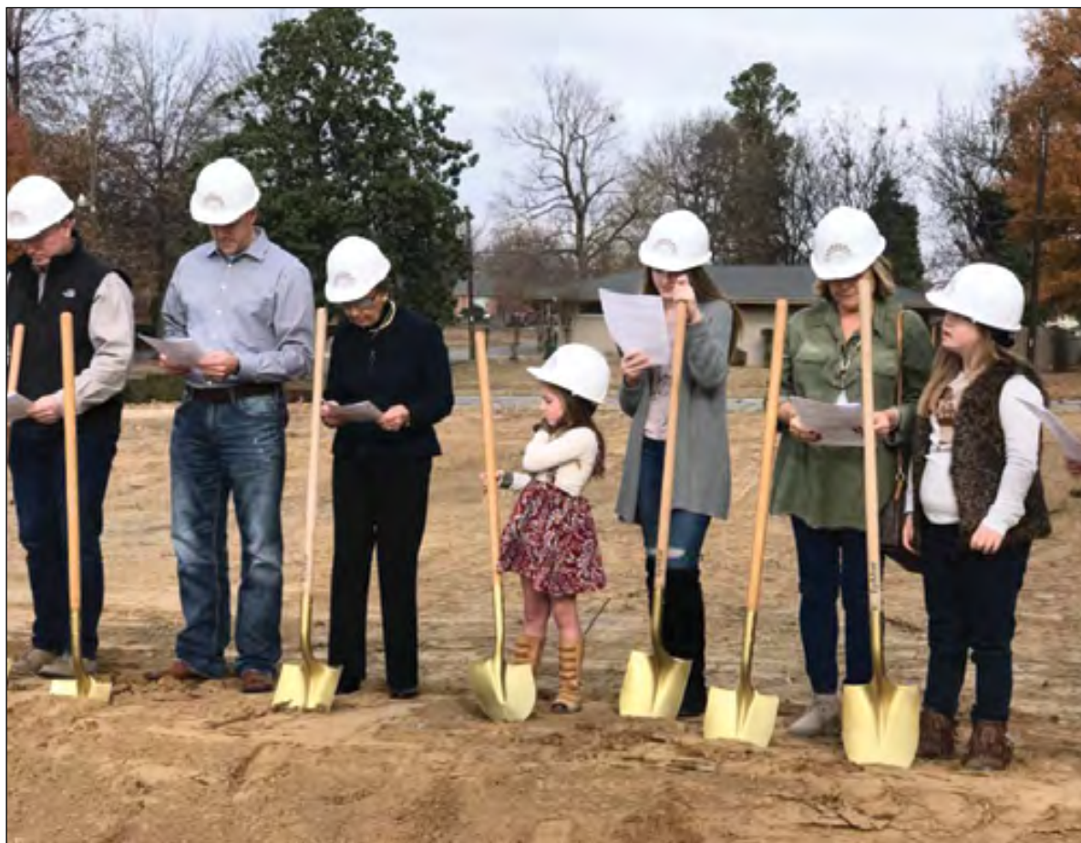
Members of Paragould First UMC turn the first spades of dirt as construction on a new addition to the church begins.
