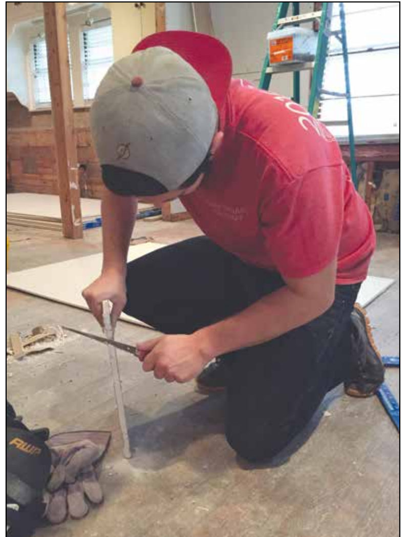
Jess Crum, a student involved in ministry with the Arkansas State Wesley Foundation, cuts a piece of drywall.
