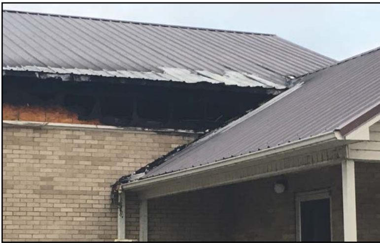
The Dec. 28 fire at Bay UMC remained hidden for quite some time, causing enough damage to the interior that the sanctuary will have to be completely renovated.
