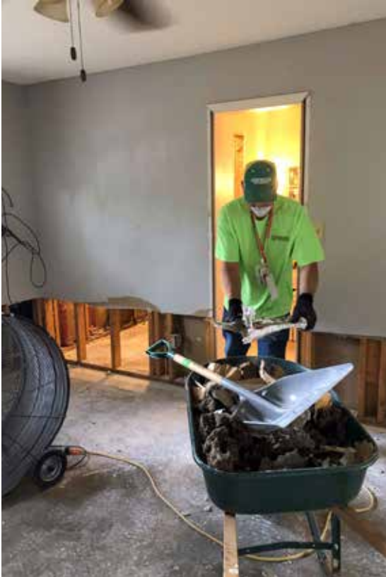
Volunteers with the Arkansas Conference Disaster Response team “muck out” the home of Keith Reeves in Fort Smith. The carpet, as well as soggy portions of the sheet rock, must be torn out and thrown away before repairs can occur. || Photo by Christina Choh
