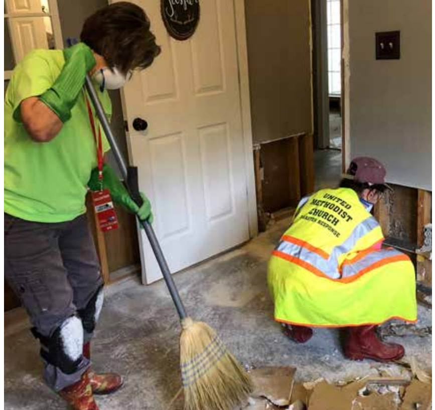
Volunteers with the Arkansas Conference Disaster Response team “muck out” the home of Keith Reeves in Fort Smith. The carpet, as well as soggy portions of the sheet rock, must be torn out and thrown away before repairs can occur. || Photo by Christina Choh
