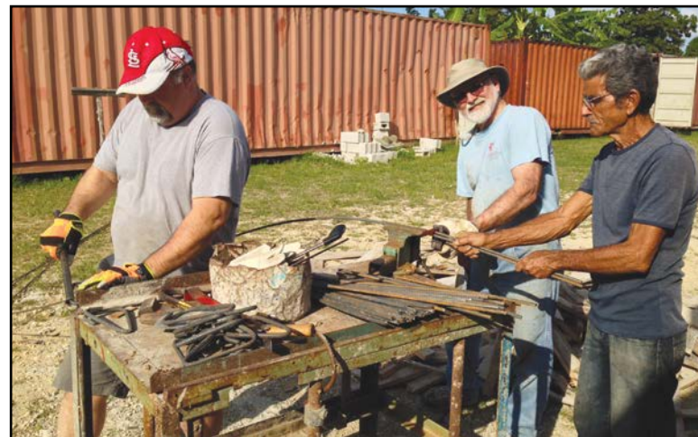
Tom Straight of Salem UMC Conway, the Rev. Chris Cooper of First UMC Little Rock and a Cuban worker trim and bend reinforcement bar for the concrete portions of faculty housing for Seminario Evangélico Metodista in Havana.
