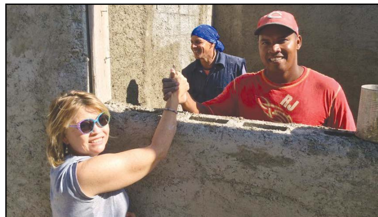
Nechi Fullerton of First UMC Little Rock and local worker Abelardo Castillo greet each other at the seminary construction site. The two met previously during a trip Fullerton made to Cuba two years ago.
