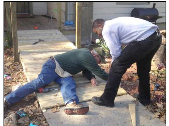
Hank Godwin, left, and BK Simmons work on a wheelchair ramp to give Simmons' sister access to her home.
