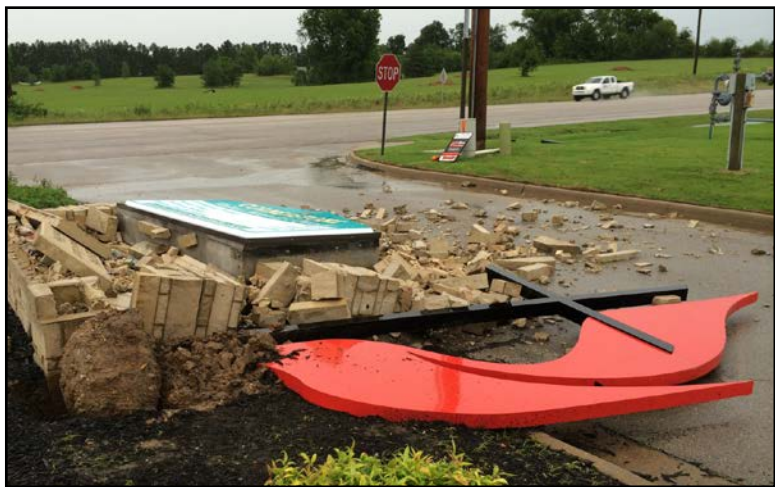
Cornerstone UMC Jonesboro sustained tornado damage to its sign (above) the same day that First UMC Jonesboro's roof was damaged, affecting music, classroom and office areas in addition to the sanctuary. Both churches are thankful there were no injuries, and repairs are in progress.
