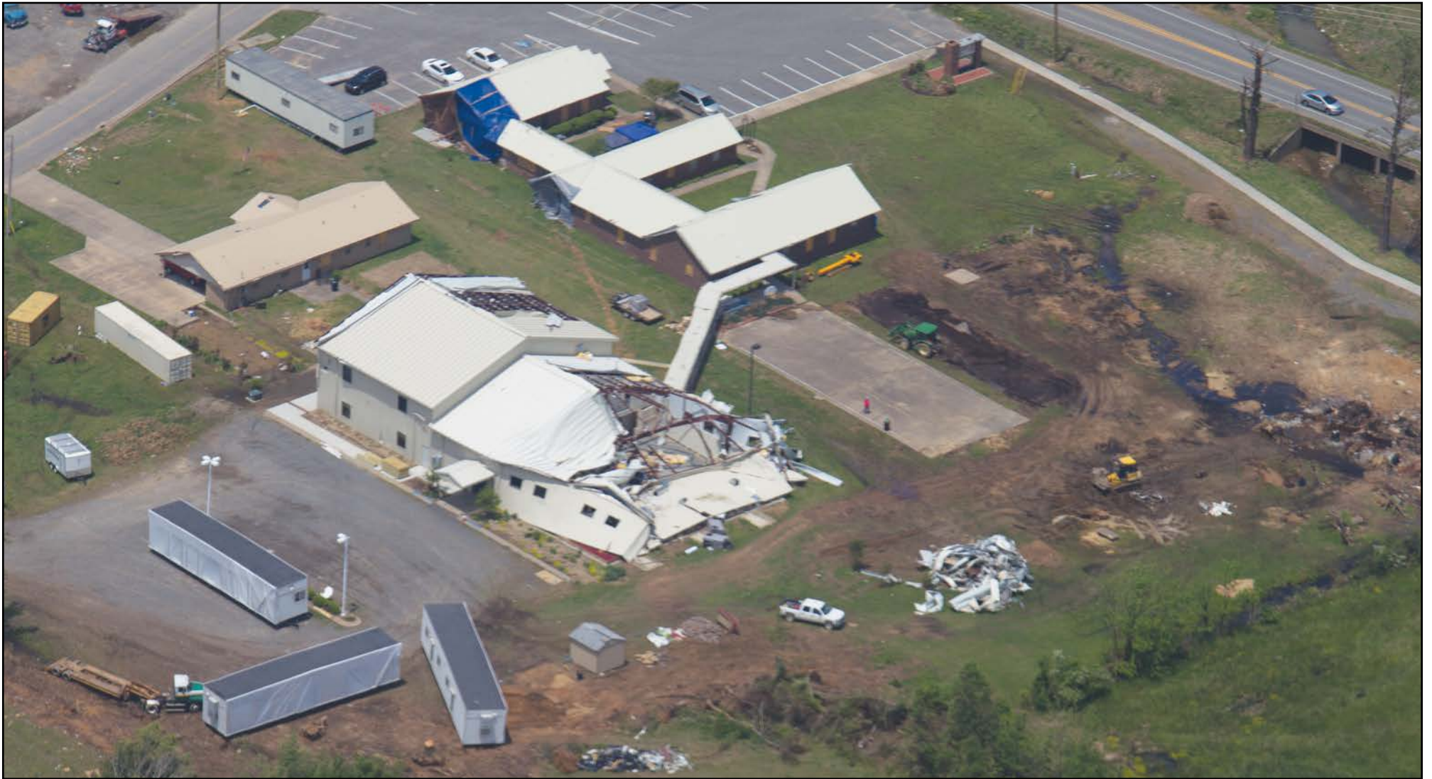
This May 19 aerial view of Vilonia UMC includes sections of a portable building (lower left) that have since been assembled for use as a temporary worship space.
