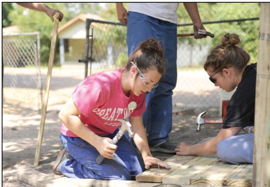
Youth work on a construction project for a neighbor during last summer's Ozark Mission Project camp in El Dorado.
