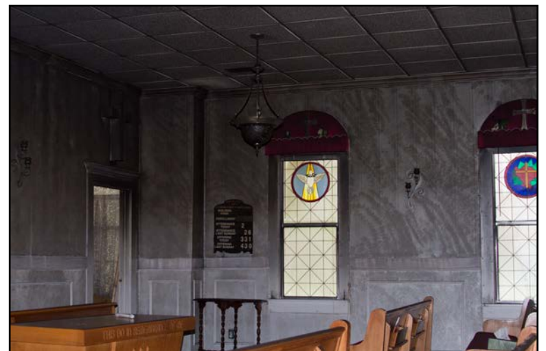
The sanctuary sustained heavy smoke damage, but was not destroyed. The fellowship hall appears to be a total loss.
