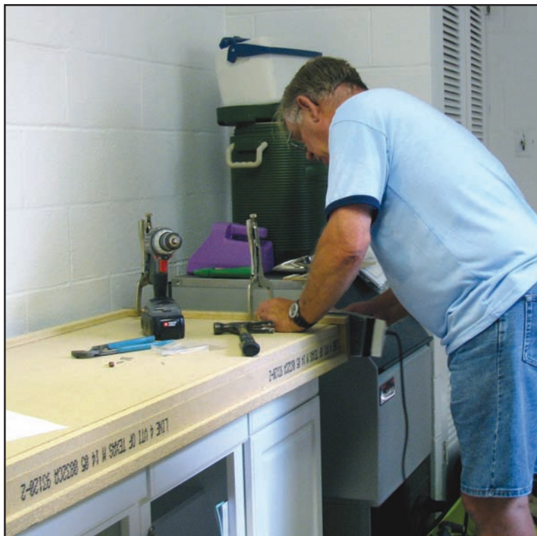
Tony Privatte, a member of Mountainside UMC Hot Springs Village, installs new cabinets and countertops at the Arkadelphia Wesley Foundation. COURTESY PHOTO
