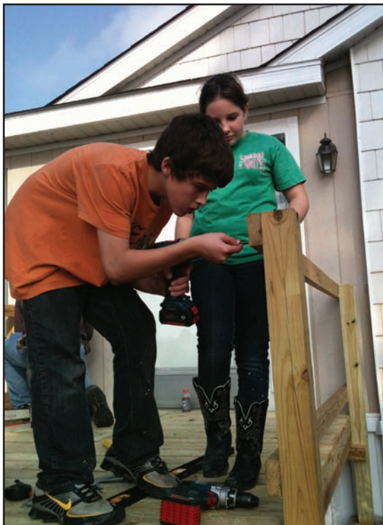
Christian O'Neal and Mallory Hudkins, members of First UMC Hope, work on the railing of the wheelchair ramp they helped build for Riley Williams and his family.
