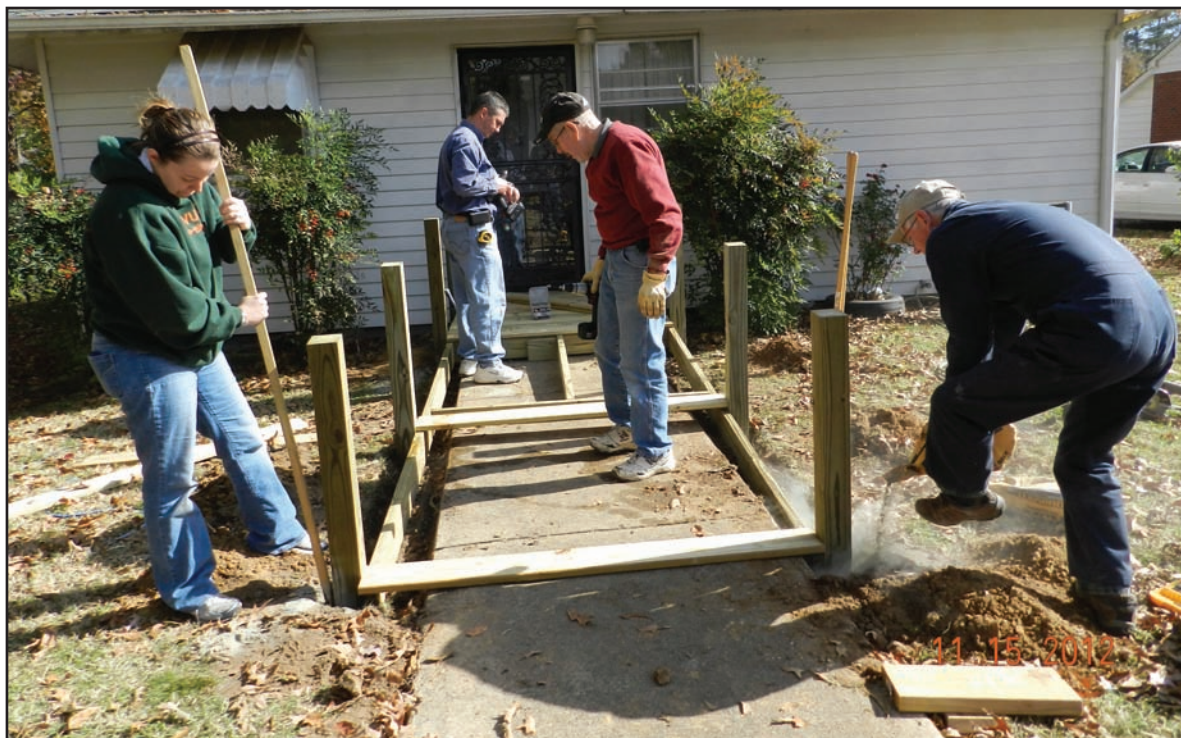
From left, the Rev. Jeanne Williams, the Rev. Chris Hemund, Bob Guelle and Brad Magee assemble the framing for a Handyman Ministry wheelchair ramp project.
