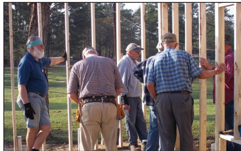
NOMADS workers frame up a new free-standing bathroom at a church camp in Texas.
