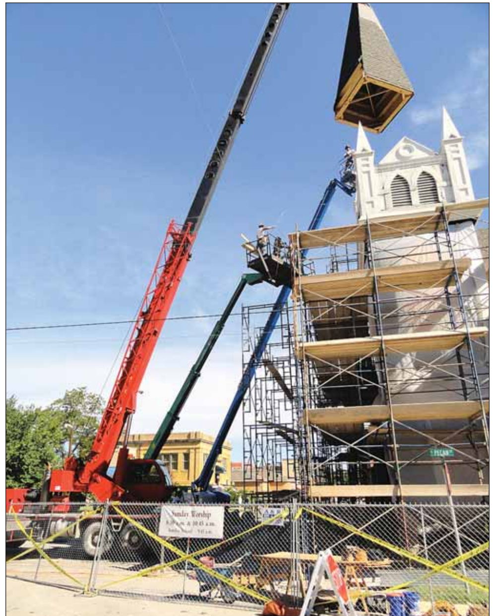
ABOVE: The exterior of the 119-year-old sanctuary building at First UMC in Gainesville, Texas, was restored at a cost of $1.2 million. BELOW: Work on the south tower steeple of the church required a crane with a 140-foot boom.
