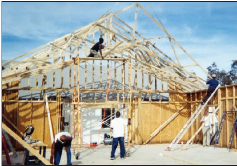
Volunteers from Theresa Hoover and St. James UMC and the Sweet Home community help build a new sanctuary for Sweet Home UMC in Pulaski County. On the ladder is Barbara Douglas, the church's pastor.
