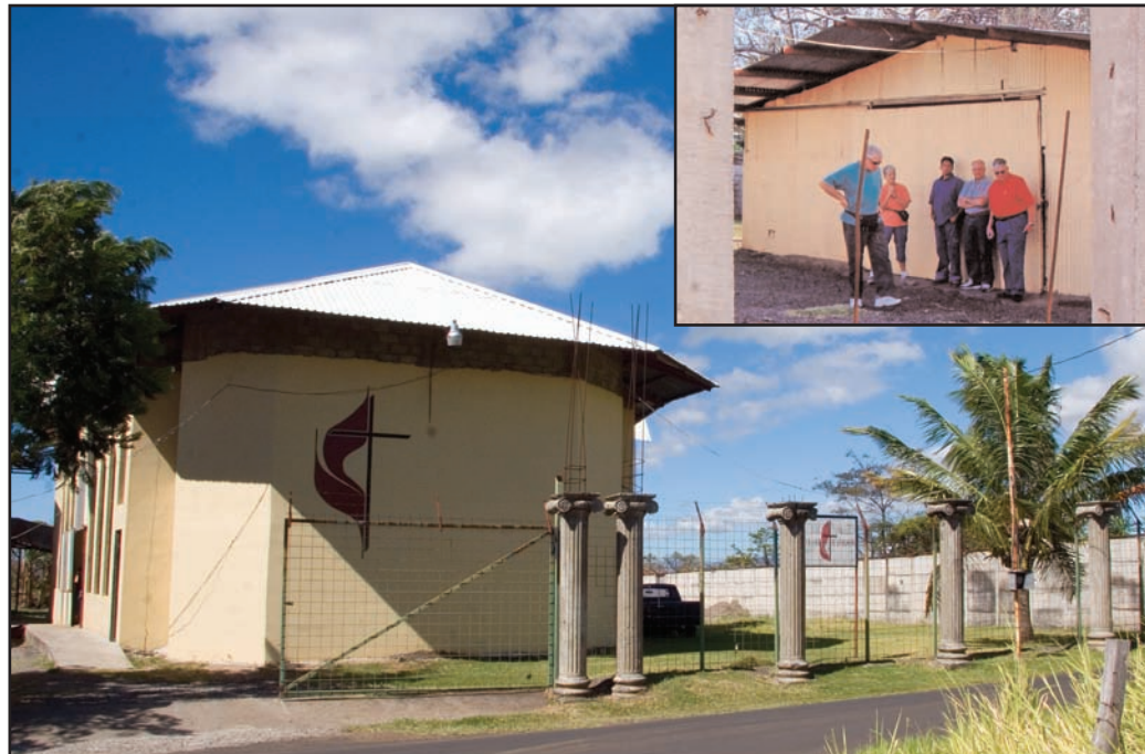
In 2004, the Arkansas United Methodist Conference's Volunteers in Mission program decided to build a new church for the congregation of La Iglesia de la Restauracion in Alajuela, Costa Rica. Since then, some 200 volunteers have worked on the project, replacing the rickety tin building shown in the inset with the two-story structure shown below.
