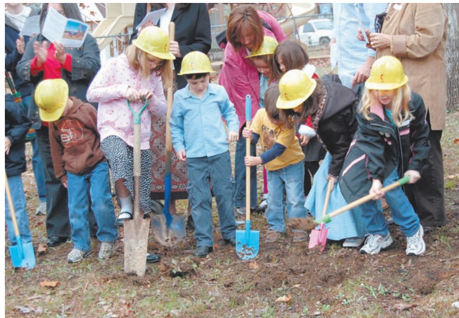
Children at Winfield UMC, Little Rock, dig in at a ground breaking for a new addition to the church.
