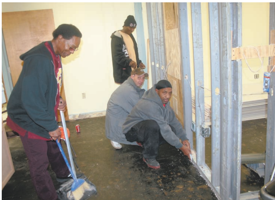
Theresa Hoover UMC members (from left) Anthony Rogers, Earnest Washington, Franklin Wagner and Shannon Dodson work to fix up the new Harmony Health Clinic in Little Rock as part of the Martin Luther King Jr. community service challenge. photo by Jane Dennis
