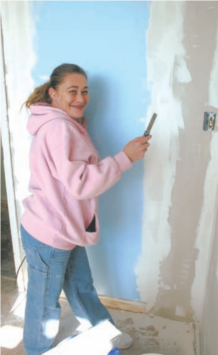
Theresa Hoover UMC volunteer Lisa Midkiff smooths the sheetrock mud in a room at Harmony Health Clinic in Little Rock.
