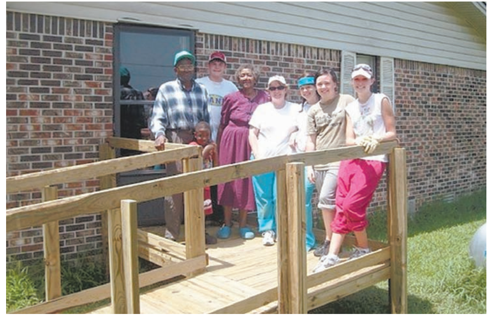
OMP volunteers along with neighbors are all smiles and very proud of a wheelchair ramp built by campers at the Cold Springs Camp.
