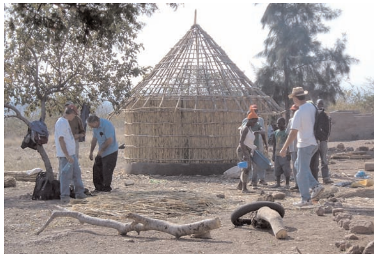
Working with Habitat for Humanity Mozambique, United Methodists from Missouri build a house July 16 in Massaca near the capital city of Maputo.
