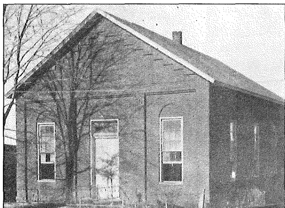
The old brick (ME, South) church on West Center Street, Fayetteville, erected in 1868.
