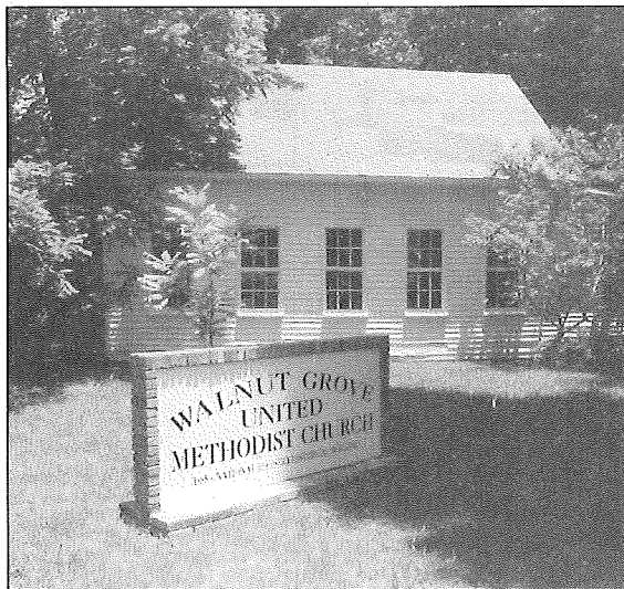
Walnut Grove United Methodist Church (Little Rock District).
