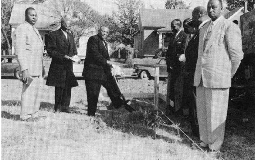
Increased church membership in the 1950s and 1960s led to the building of many new church structures. This groundbreaking ceremony for a new parsonage at Mallalieu Church in Fort Smith is typical of the ceremony held in many places. The Rev. C. C. Hall is holding the shovel and behind him is the Rev. B. F. Neal.
